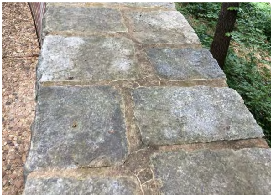
SALVAGED GRANITE CAPSTONE
